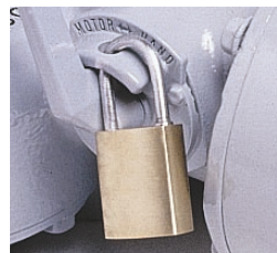
Padlockable Clutch Lever
